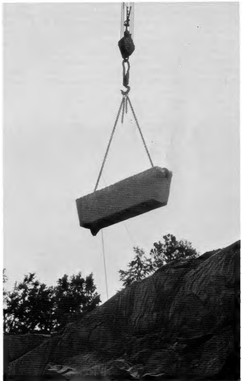
Once the massive pieces of stone were freed from the ledge mass, derricks gingerly lifted them to the rim of the quarry as shown above. Quarrymen were especially wary in this phase, since the derricks normally don't lift such extreme weights.
